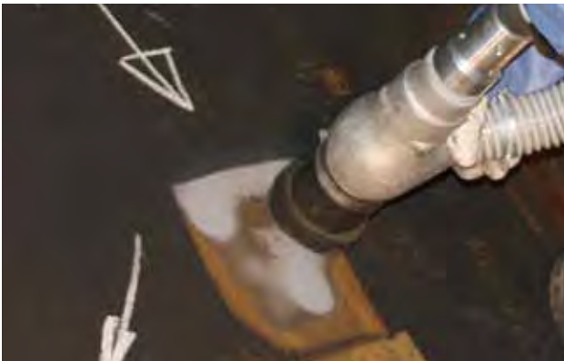
Cleans structures and removes harmful isocyanates that are released during welding and heating
