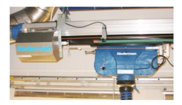
The trolley return unit is very suitable for high capacity drive through applications, e.g. vehicle inspection centers and bus garages etc.
