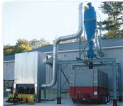
Cyclone with NFP after-filter
