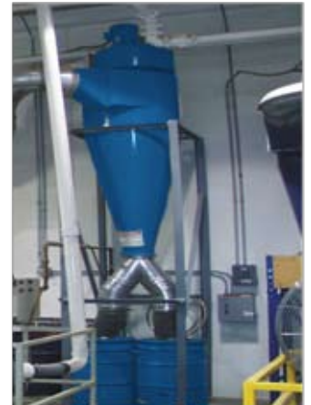
Barrell Loading Structure
